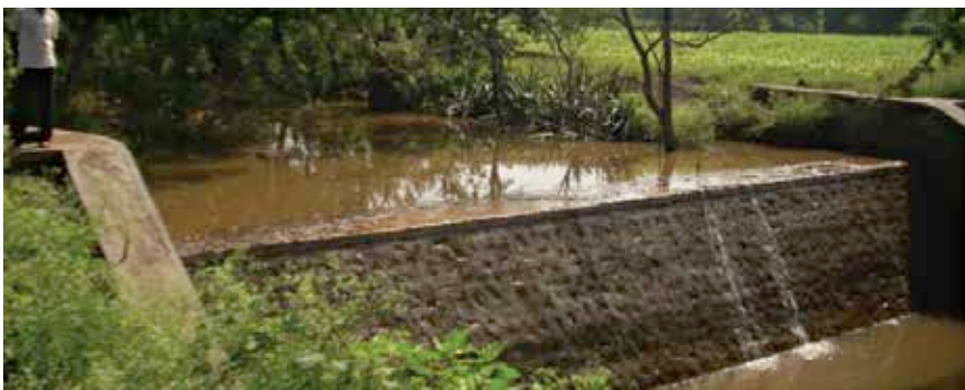
A check dam restored by JBGVS
