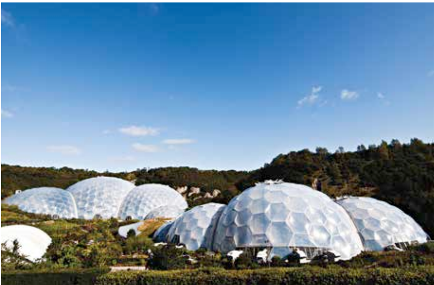
The Eden Project features hexagonal tiles made of polymer that allow plenty of natural light into the conservatories. The hexagonal pattern is one example of biomimicry
