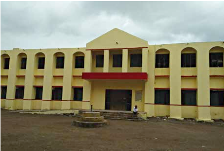
Newly painted school at Ranjangaon
