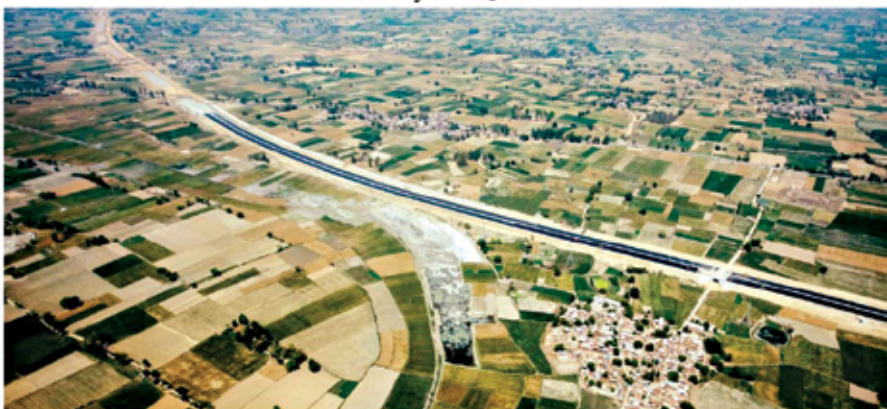
An aerial view of the Unnao - Kannauj stretch of the Agra Lucknow expressway nearing completion
